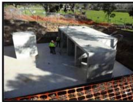
Concrete storage tank during construction
