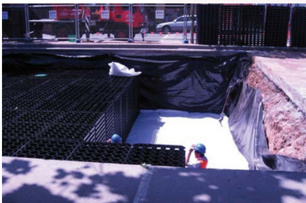
Underground storage tank under construction (Image courtesy of Spiire)
