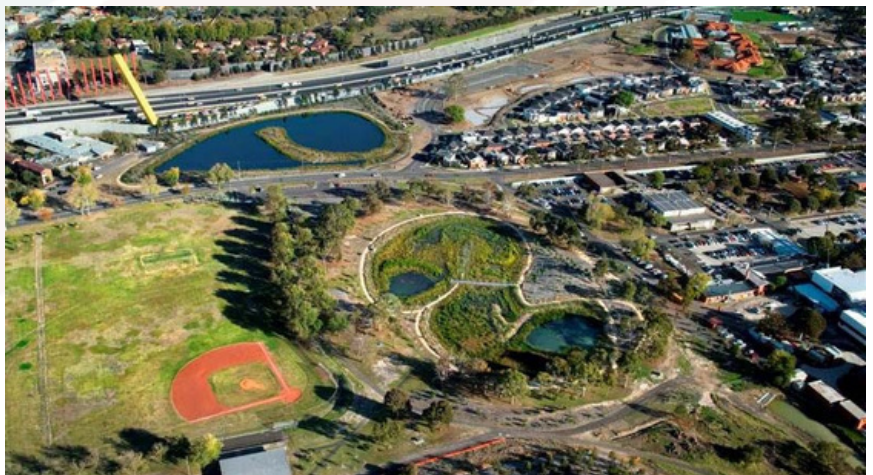
Royal Park wetland and storage basin (image courtesy of City of Melbourne)
