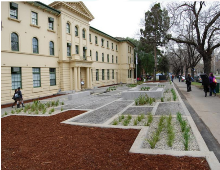
Victorian College of the Arts street frontage – Raingardens during establishment phase
