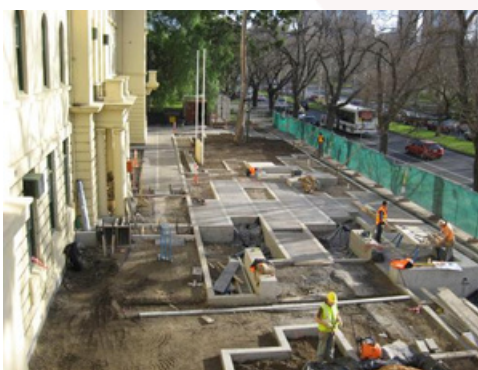
Raingardens during construction
