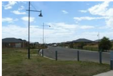
Houses nearing completion
