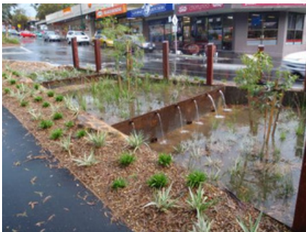
Each raingarden incorporates a tiered design approach which overcomes the site constraints posed by the very steep gradient
