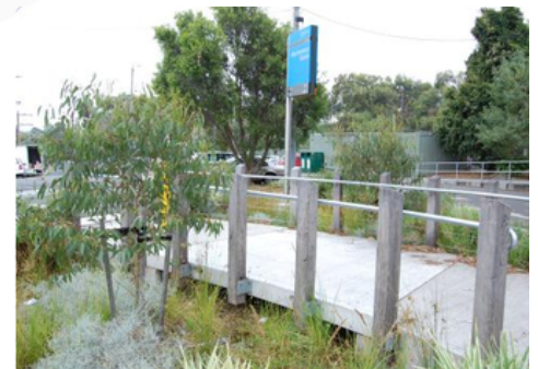
A boardwalk was installed over the raingarden to facilitate pedestrian movement
