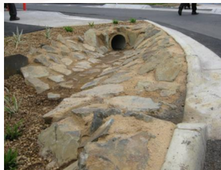
Inflows into the raingarden include catchment-wide runoff and direct street runoff
