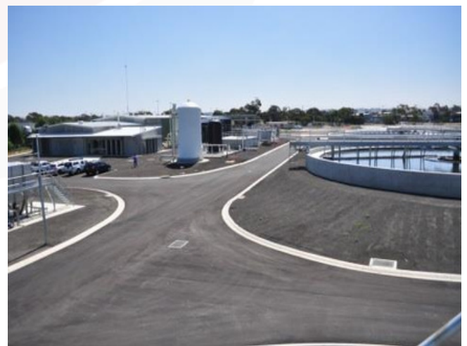
Class A recycled water from the plant has reduced demand on drinking water supplies and its reuse supports the State Government's reform for integrated water management.
