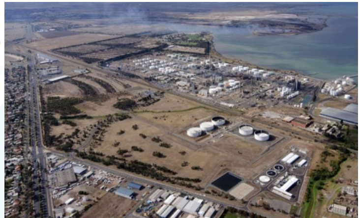
The Northern Water Plant (bottom right hand corner) and Viva Energy Geelong Refinery from the air.
