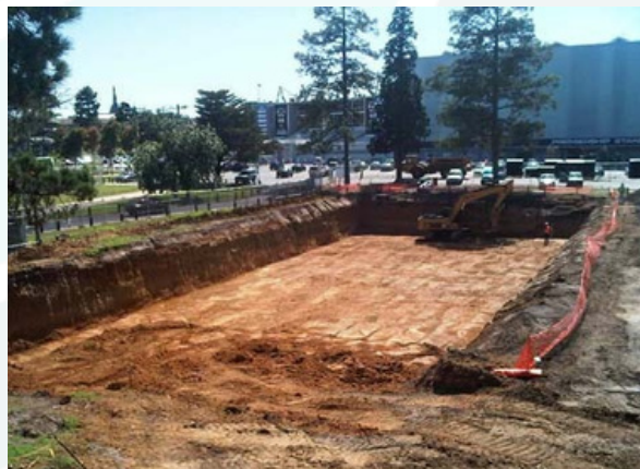
Kardinia Park, Stormwater Harvesting Project – Construction of underground storage tank
