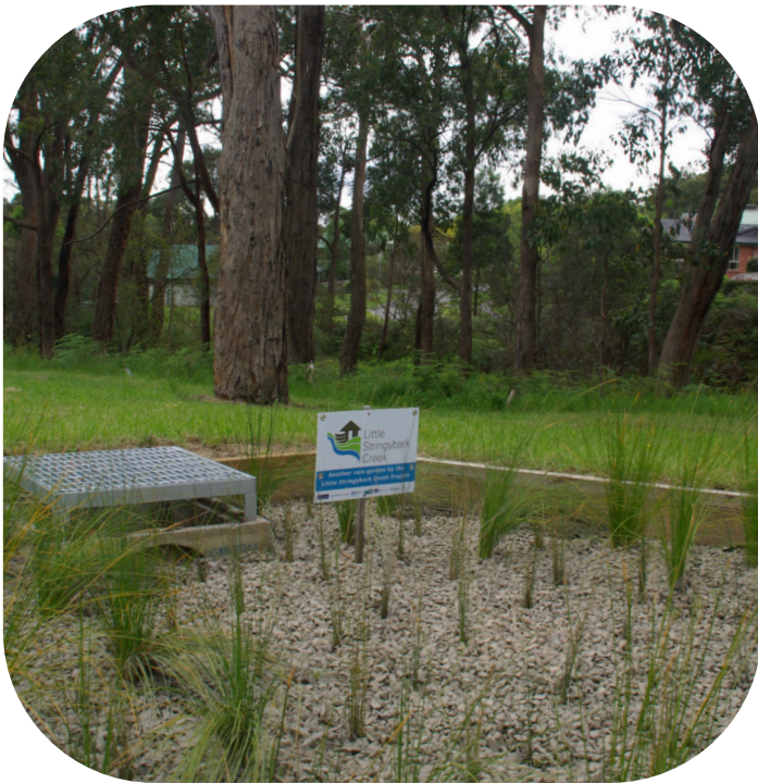
Infiltration Rain Garden, Mount Evelyn
