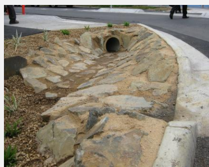
Inflows into the raingarden include catchment-wide runoff and direct street runoff
