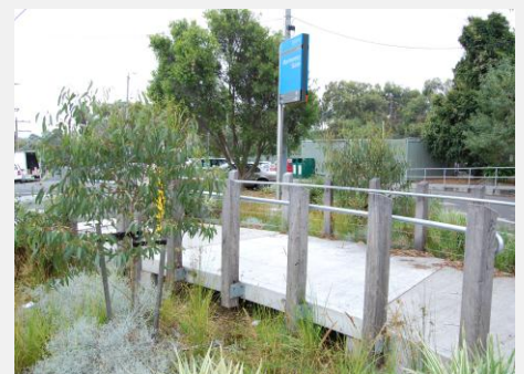
A boardwalk was installed over the raingarden to facilitate pedestrian movement
