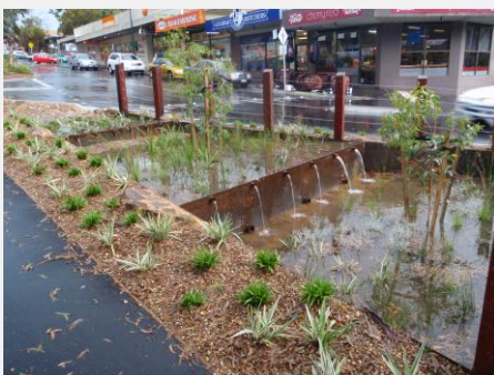
Each raingarden incorporates a tiered design approach which overcomes the site constraints posed by the very steep gradient
