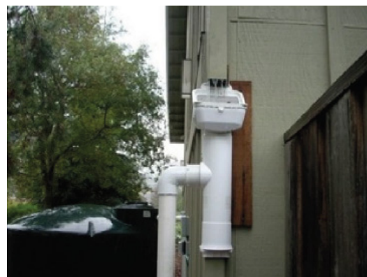
Figure 8. A tank set up with a first flush diverter at the wall
