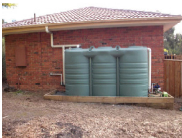
Figure1. Rainwater tanks collecting water from the roof
