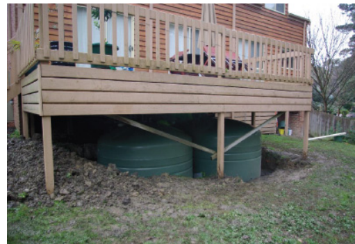
Figure 6. Dual tanks underneath a deck and partially underground. A great example of maximizing space available and reducing excavation
