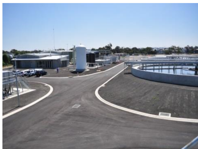
Class A recycled water from the plant has reduced demand on drinking water supplies and its reuse supports the State Government's reform for integrated water management.
