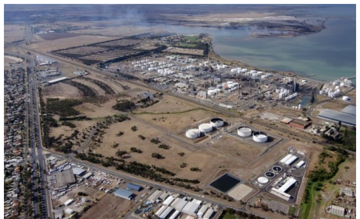
The Northern Water Plant (bottom right hand corner) and Viva Energy Geelong Refinery from the air.
