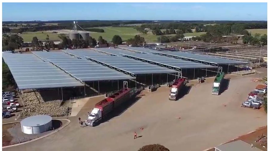
Roof water harvesting provides a sustainable water supply for truck washing at the Hamilton Regional Livestock Exchange (Photo Credit: Central Steel Build http://www.centralbuild.com.au )
