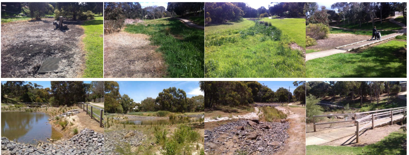
Jan Juc Creek Daylighting Stage 1 before (top) and after (bottom) photos.
