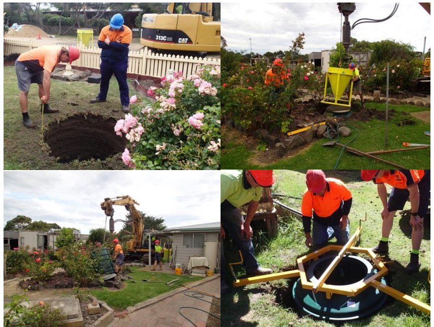
Installing a pressure sewer system for Poowong Loch & Nyora Sewerage Scheme
