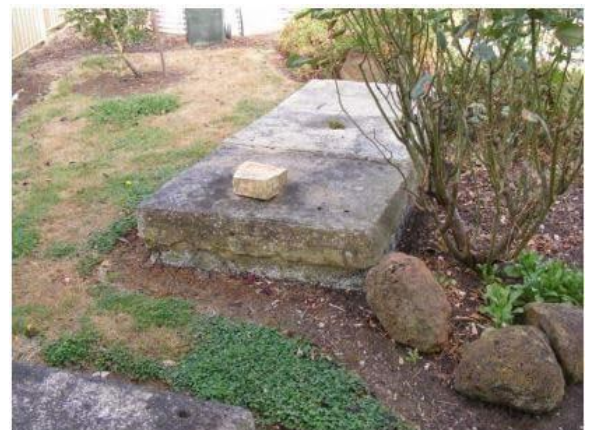
A black water septic system in the township of Branhholme.
