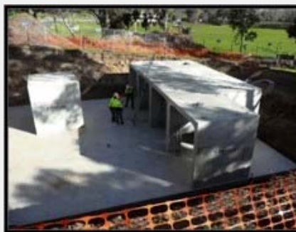
Concrete storage tank during construction
