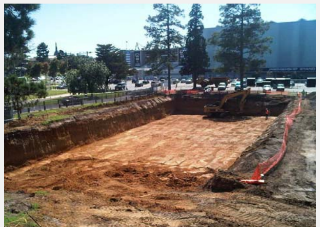
Kardinia Park, Stormwater Harvesting Project – Construction of underground storage tank
