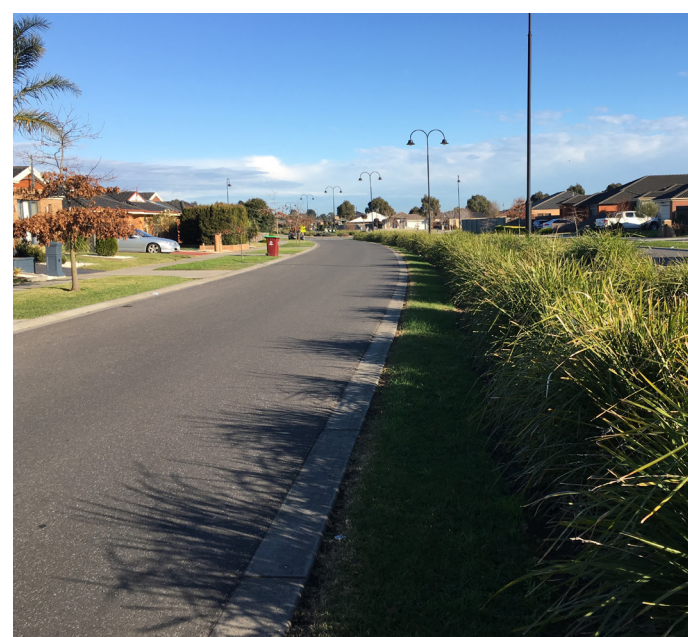
An example of a water stormwater asset in the City of Casey
