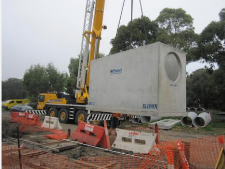
Two large gross pollutant traps allow material to be captured before the water enters the storage area.
