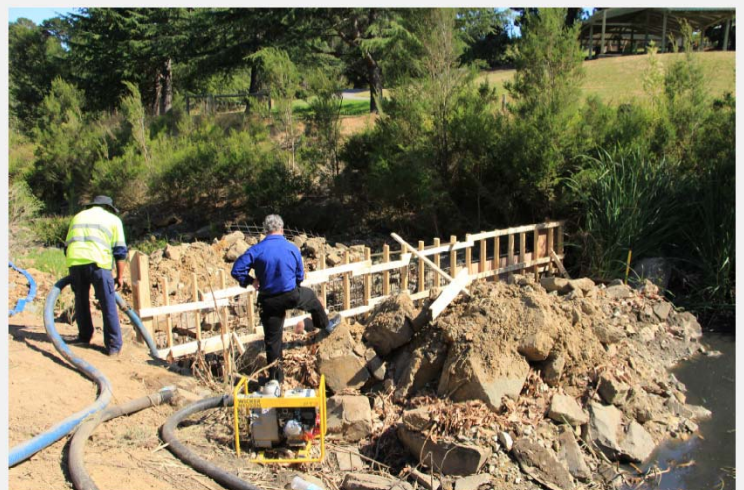
Weir construction in Ruffey Creek
