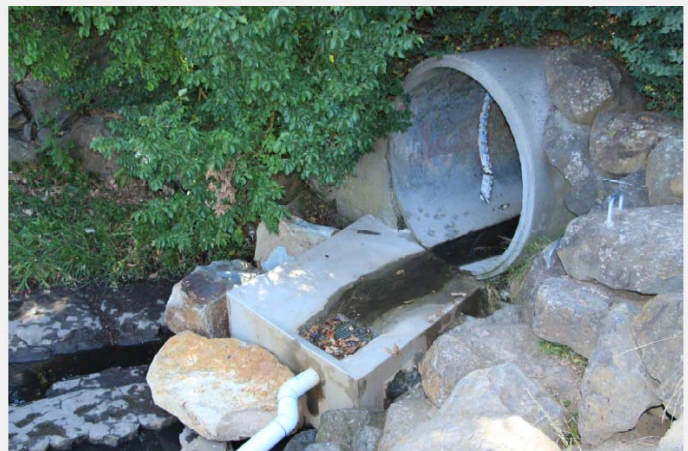
Diversion structure to maintain environmental flows in Ruffey Creek
