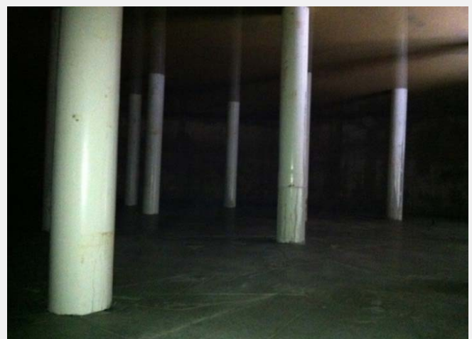
Inside the underground storage tank
