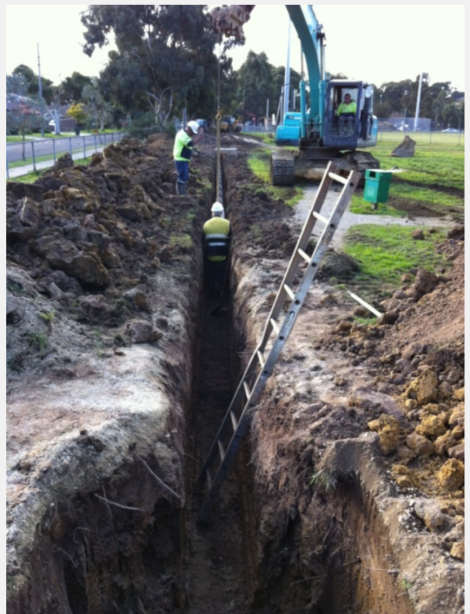
Installing the diversion pipeline
