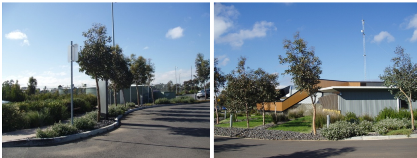
Figure 9 Craigieburn Health Services (right) and storage tanks for fire hydrant water (left).
