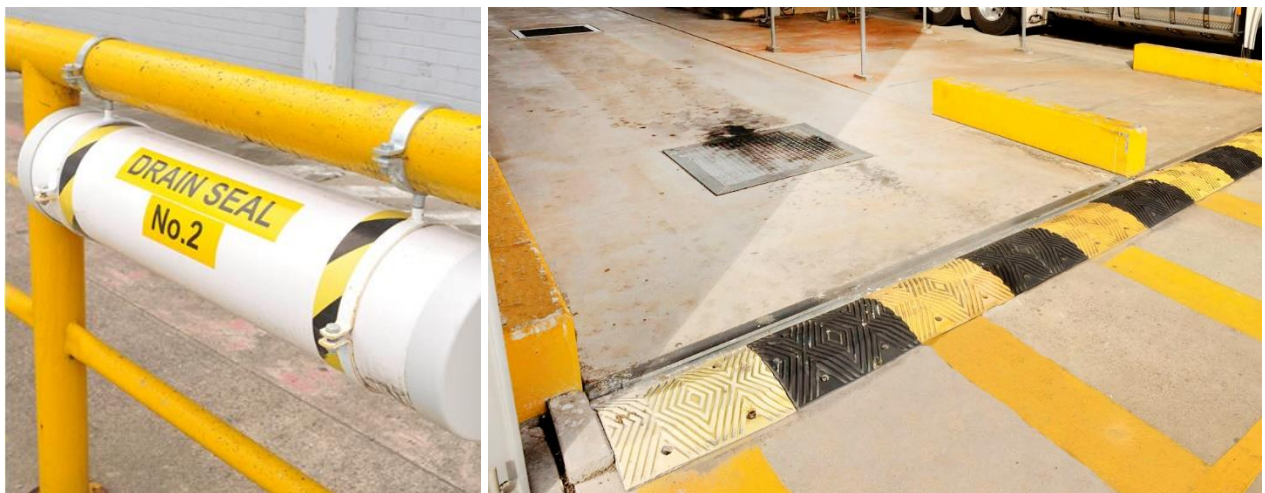
Figure 7.5. Drain seal (left) and rollover bund (right).
