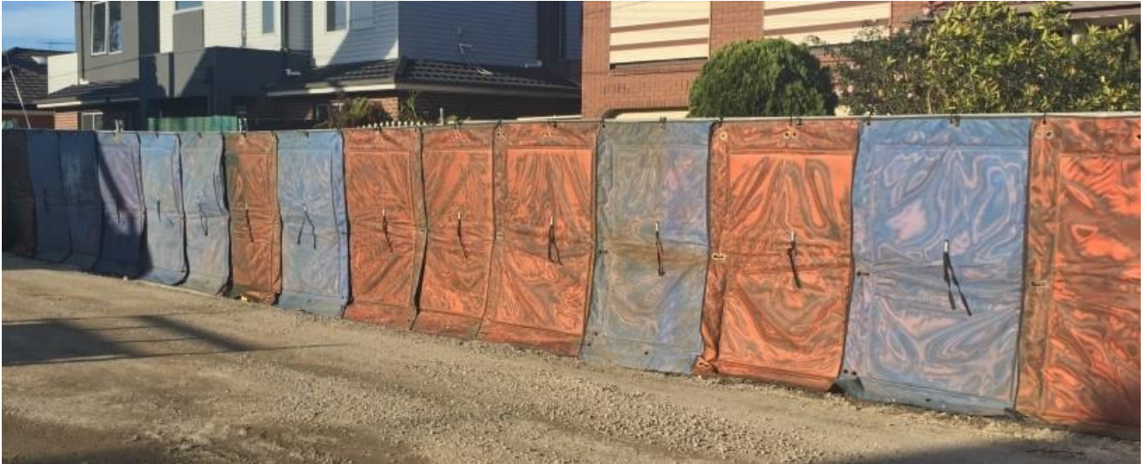
Figure 4.3. Temporary noise barrier. (photo courtesy of John Holland)
