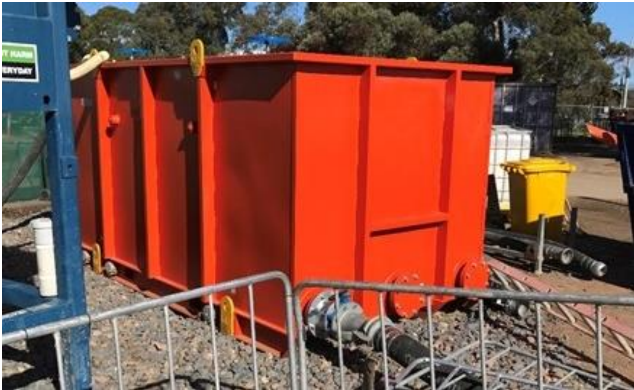
Figure 5.2. Portable sedimentation tank. (photo courtesy of McConnell Dowell)
