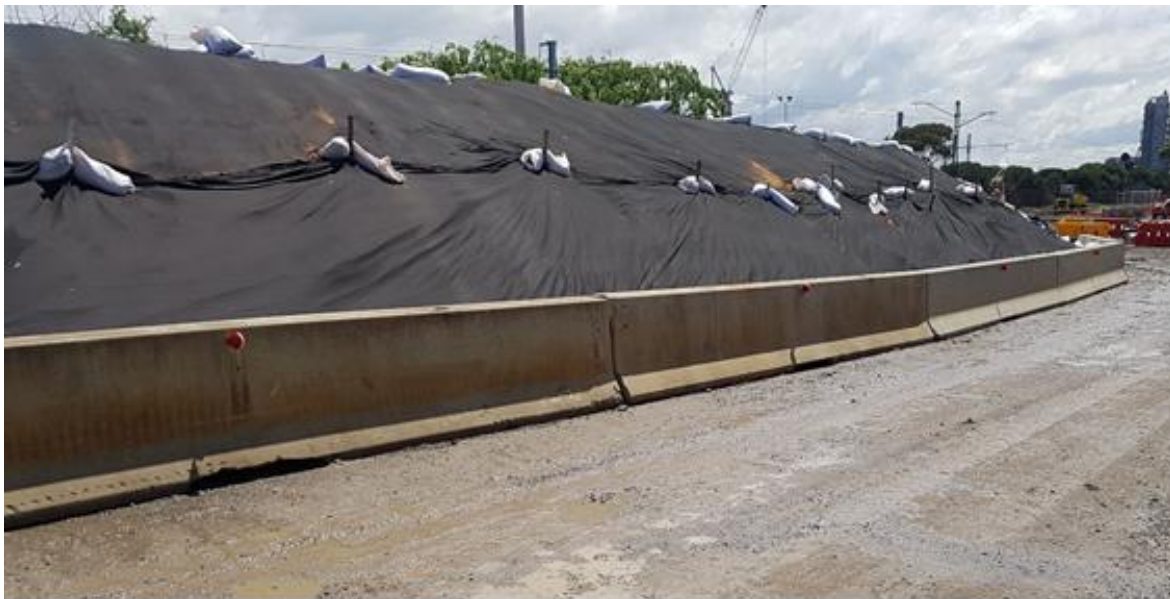
Figure 2. Covered stockpile. (photo courtesy of McConnell Dowell)
