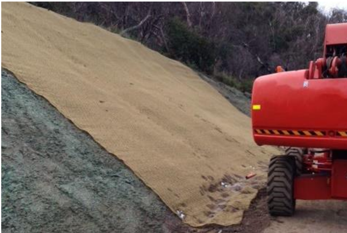
Figure 5.1. Slope stabilisation controls. (photo courtesy of Regional Roads Victoria)
