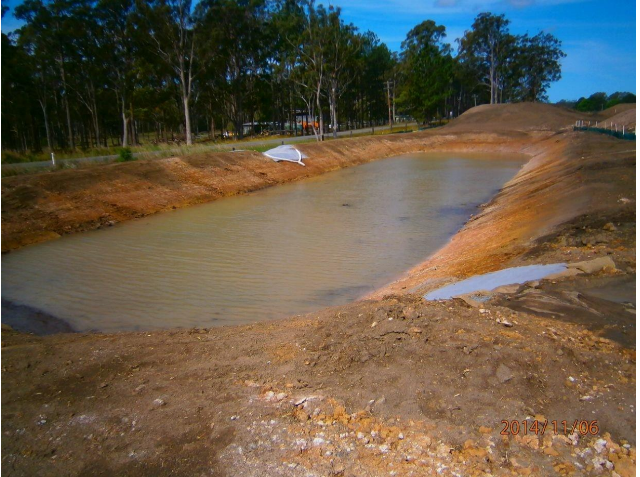
Figure 5.4. Installed sediment basin. (photo courtesy of McConnell Dowell)
