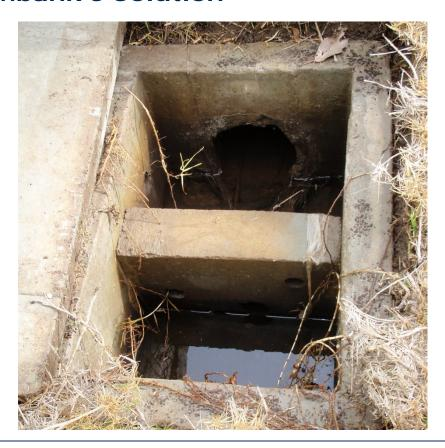
We visited a second wetland to see its outlet structure: an orifice plate controlling the flow of water from the wetland
