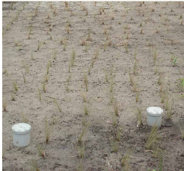
Figure 7 Example of inspection openings in a raingarden
