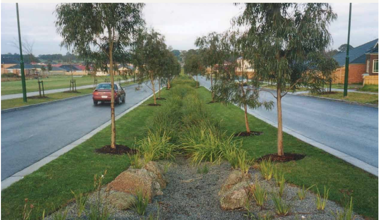
Figure 13 Example swale (photo source: wsud.org.au)
