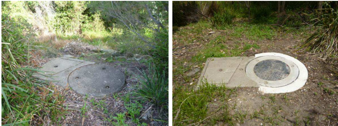
Figure 20 All Cleansall 375 GPTs need the lids replaced with ones that can be opened for inspection and cleaning without the need for a machine. Photos above show a CleansAll 375 lid before, and after, which also included a new lid surround, to prevent the dirt falling in when the lid was removed for cleaning.
