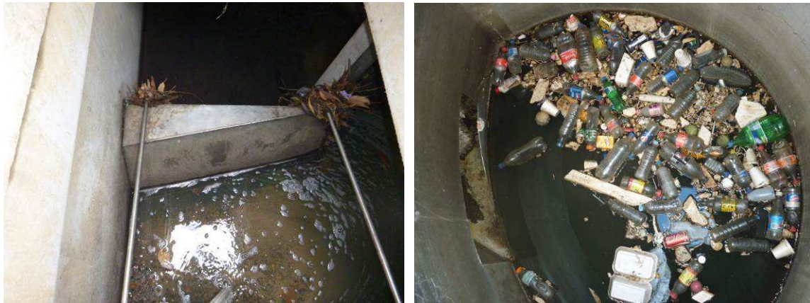
Figure 10 The Humegard weir has bent, is wedged in a low flow bypass position and flow is going over the boom that could not handle the force of the water due to the high grade and velocity of the incoming flow. The VortCapture GPT is a vortex style device designed to utilise the energy in higher velocity flows.
