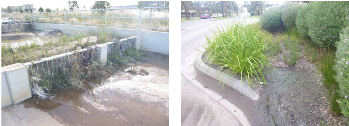
Figure 17 In this photo, the developer has shown pure neglect for the trashrack. This is disgraceful. And a raingarden so overloaded its stopped working.
