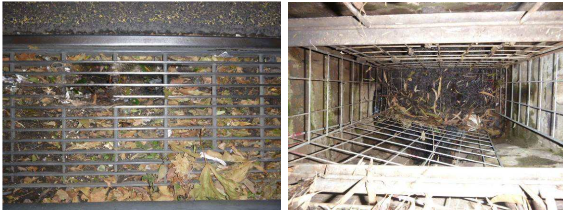
Figure 15 Full to ground level and no flow going through the pit. No bag, frame broken, frame extends over the pipe at the base, so there is nothing good about this trap.
