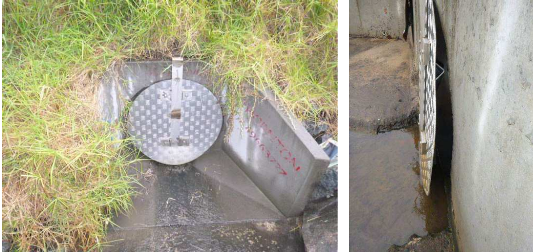
Figure 18 Most tidal flaps get bent and don't seal, so they don't stop the tide anyway.
