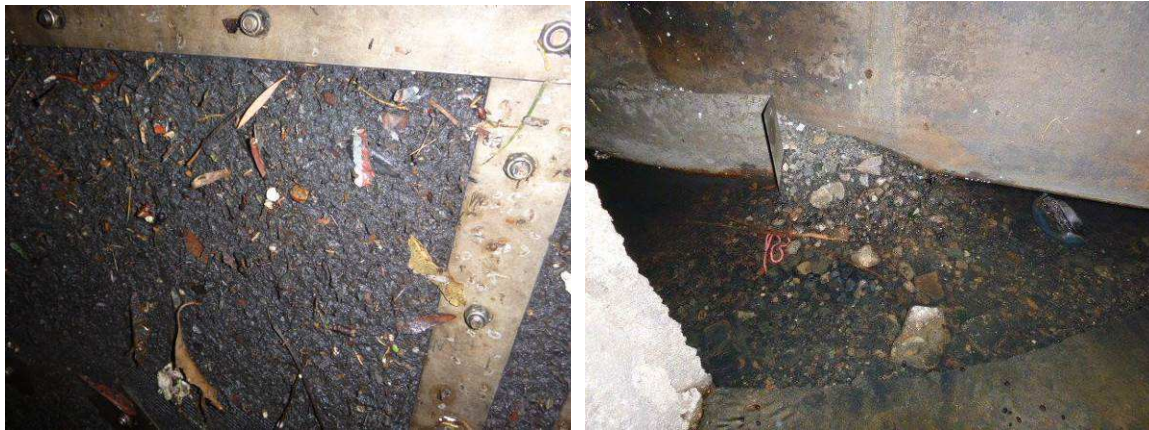
Figure 12 Blocked screens. Sediment buildup behind the screens.
