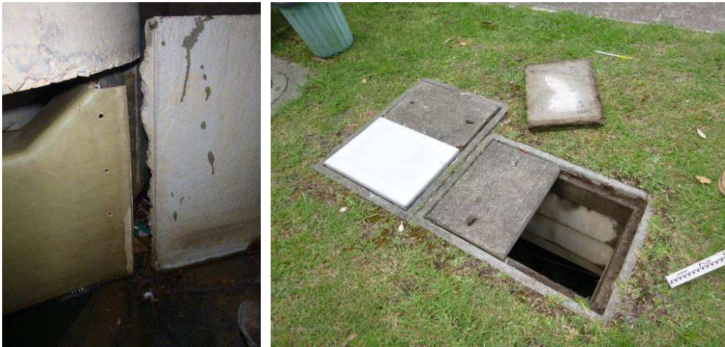
Figure 7 The precast weir in a completely standard CDS unit was installed back to front so the inlet chute attaches to nothing and there is a 50mm gap between the weir and the inlet. In the photo on the right, the Humegard lid was put on 90° wrong, so there is no vertical access to the screens or pollution storage zone. Poor installation and no inspection at handover.
