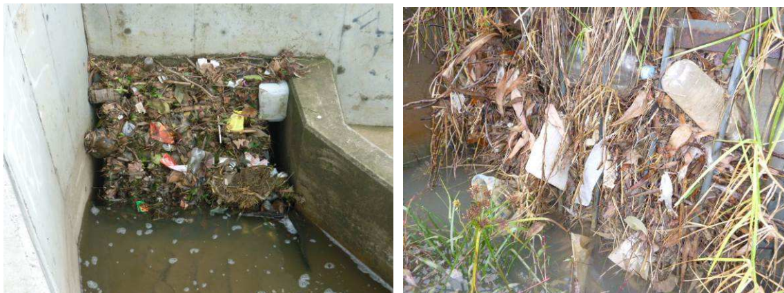
Figure 8 Inlet exclusion bars with poor design. Outlet exclusion bars with poor design. Poorly considered exclusion bars lead to blockage, bypassing, pollution downstream and high maintenance costs.
