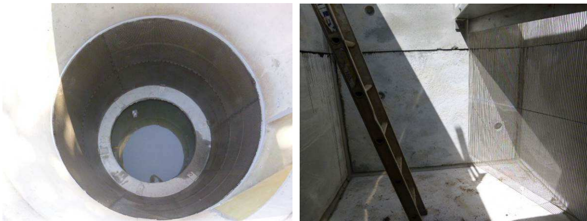
Figure 4 The sump storage volume is more important than performance. CDS units and Humegards have generally large storage volumes.
