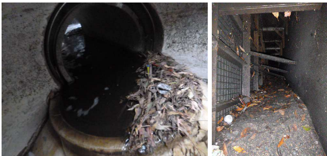
Figure 3. Humeceptor inlet blocked, but not on the cleaning spec to check it or clean it. Sediment buildup behind Ecosol screens without the specification to clean behind the screens.
