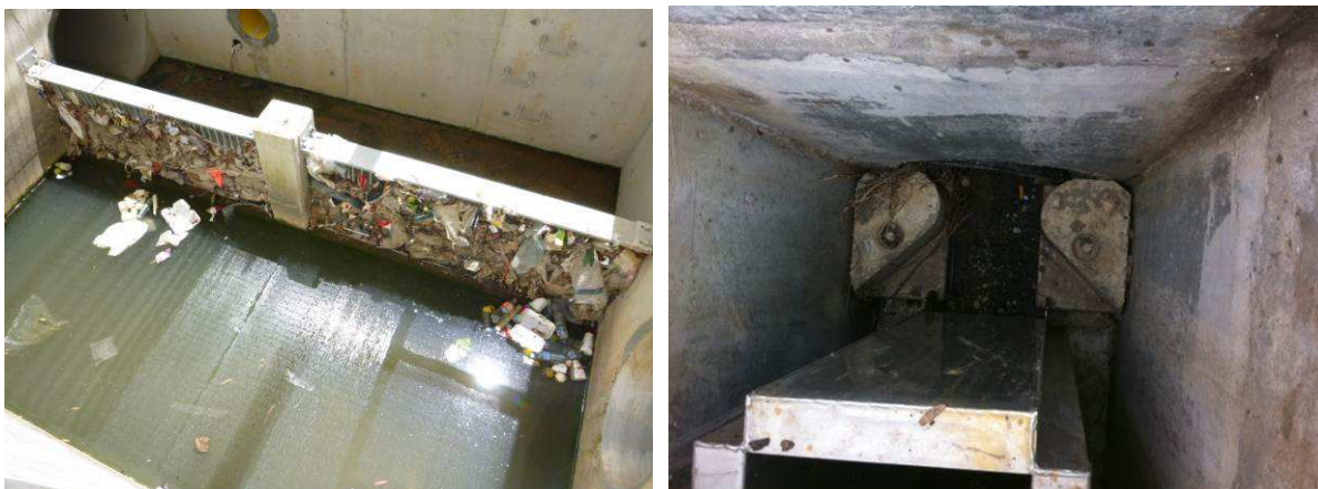
Figure 5 For the pipe size and catchment area, this trashrack is way too small. For the catchment this Ecosol was way too small, its structure is half covering the inlet pipe and was very quickly full and non-operational.
