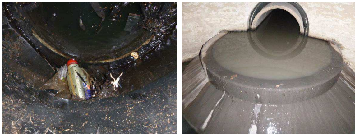
Figure 13 Blocked inlets and more blocked inlets.
