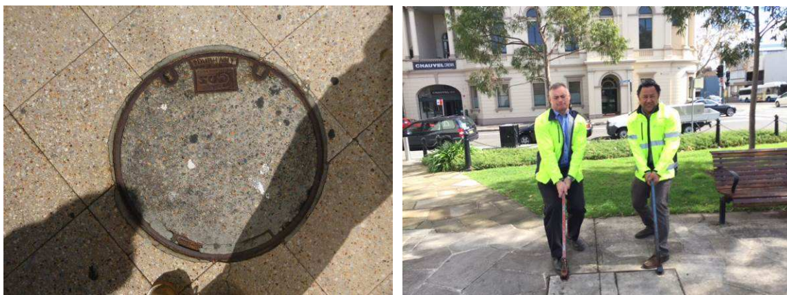
Figure 11 The CDS diversion chamber was not opened for so long that is now has to be replaced. Larger lids, especially heavy duty gatics become a real WHS issue over time, and really need to be greased EVERY year or even 2 men wont be able to open them.
