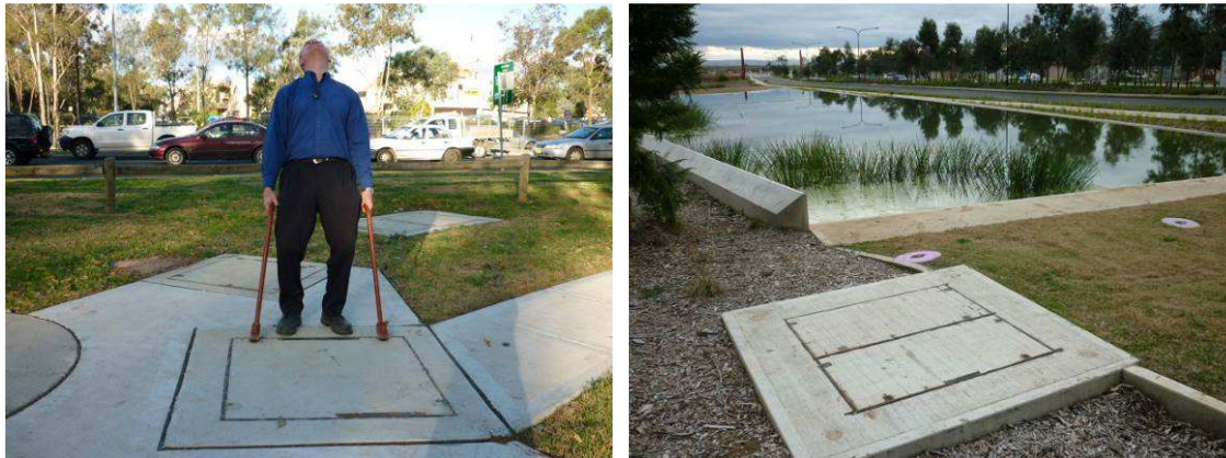
Figure 19 If there is the need for large lids, make them 2 part. Don't automatically go for D class lids if you are not putting them in a roadway. The easier it is to monitor and clean your SQID assets, the more reliably they will get cleaned.
