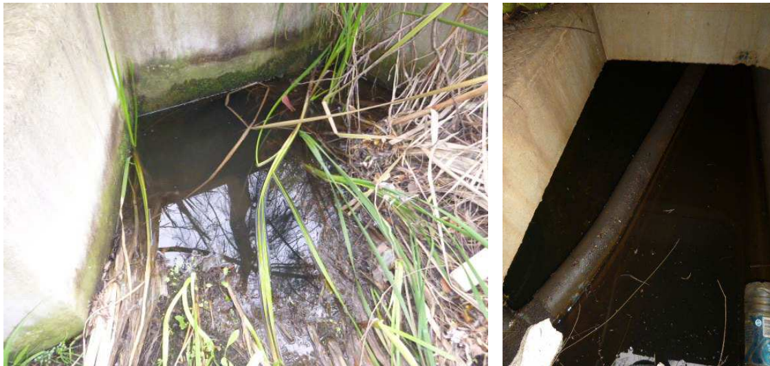
Figure 6 Elevated downstream creek levels have caused the pipe to be completely submerged, and the CleansAll weir that should be 600mm tall is only 30mm high. Non-operational.
