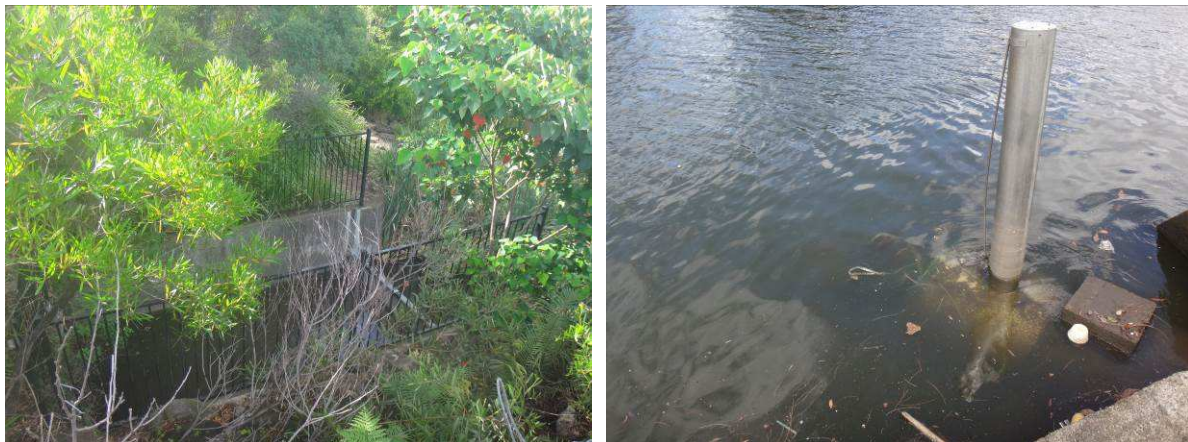
Figure 9 This GPT has no vehicle access, so manual cleaning is required, and this results in higher costs and lower performance. The submerged nettech above requires cleaning contractors to drive across a golf course to access it. Poor hydraulically, poor access.
