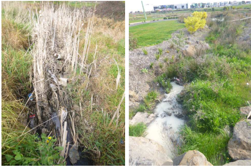
Figure 16 Vegetated swale with pollution and grass swale with paint spills.
