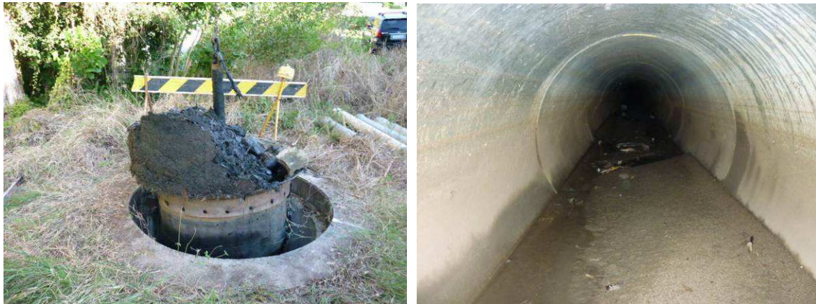
Figure 2 A basket massively overfull. A forgotten GPT leads to deposition in the upstream pipe and potential flooding issues.
