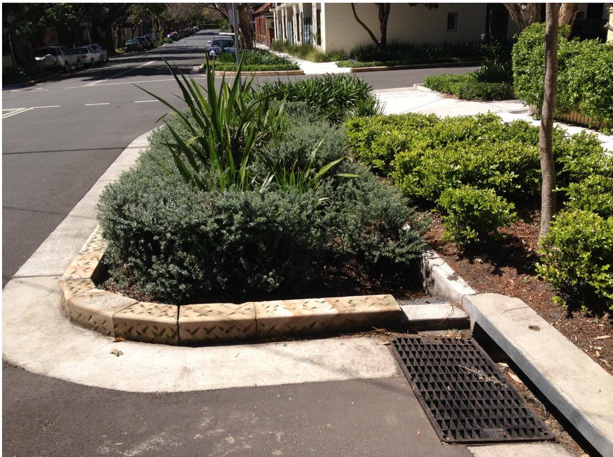
**Photo 1: The raingarden at Telopea Street with an entry pit.**
