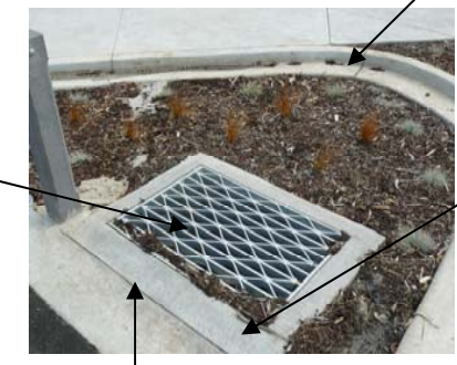
Avoid use of organic mulch on top as material floats and block drain
