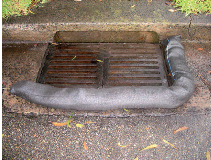
Figure 2. Filter sock installation
