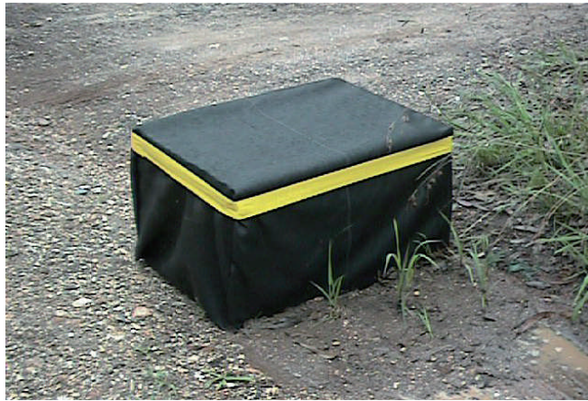
Figure 3. Filter Bale installation
