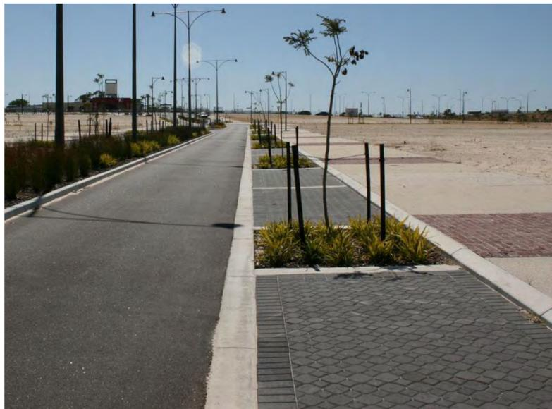
PHOTO EXAMPLE OF TYPICAL BRICK PAVING WITH BIO FILTRATION POCKETS OR RAINGARDEN
