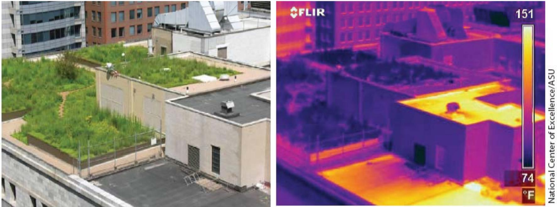
On a typical day, the Chicago City Hall green roof measures almost 80°F (40°C) cooler than the neighboring conventional roof.
