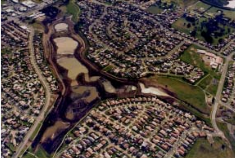
Large scale constructed wetlands in Melbourne, Victoria.
