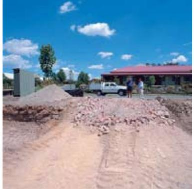
The entry/exit pad should extend from the kerb or road reserve to the building slab, and where it slopes toward the road, a hump should be installed across the pad to deflect stormwater runoff.
