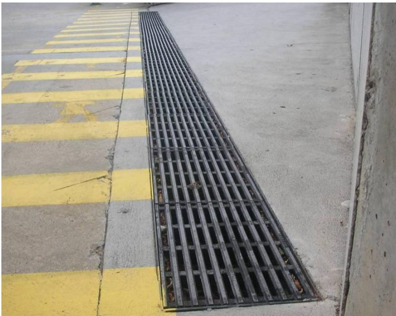
Figure 7. Example of a trench grate
