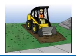
Remove a 3m or greater strip of soil from road (or where concrete crossover ends) to nearest building point or a minimum of 5 m.
