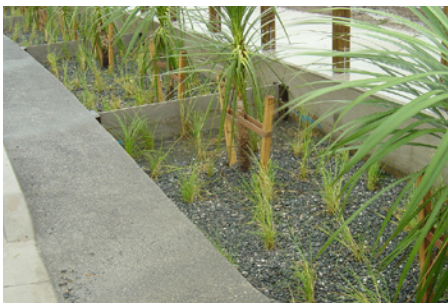
Rain Garden at Albany Park and Ride station - finished rain garden
