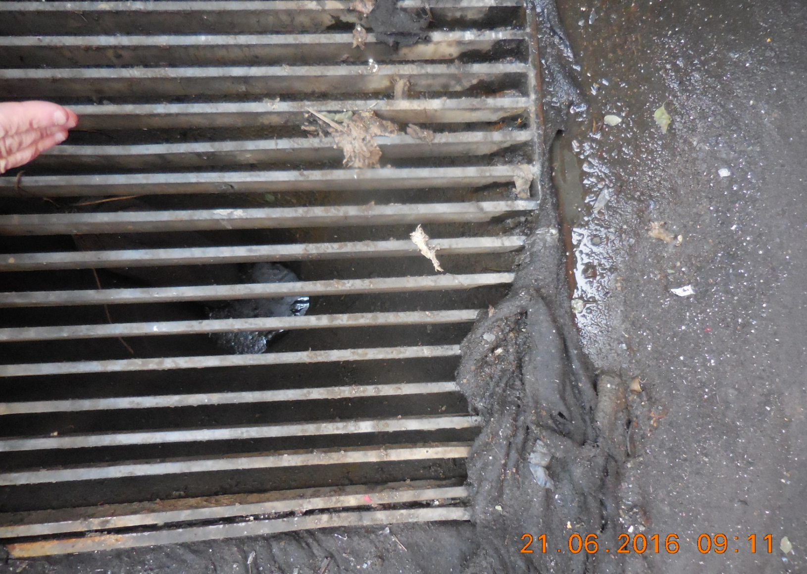
Stormwater pit adjacent engine dismantling bay. Sediment sock installed. Heavily soaked in waste oil.
