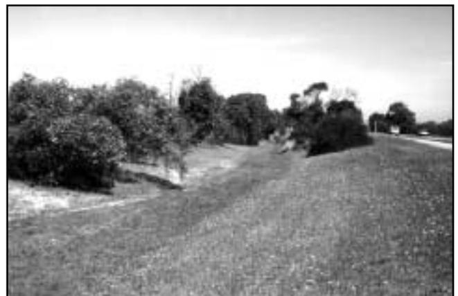
Figure 5.3 Swale drain along the side of highways is an effective means of treating stormwater runoff.
