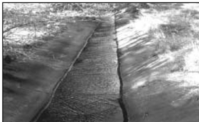
Figure 2.5 Urban waterways are often channelised and concreted to improve hydraulic efficiency
