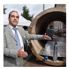
A medium to large sewer (900mm or larger) with constant flow (12 litres/second or more) is required within close proximity (<150m) to the heating/cooling demand. Renewable/clean energy grants or rebates would offset capital cost but are not critical.
