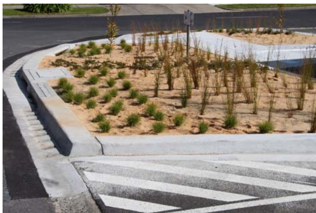
Highview Drive, Doncaster, vegetated ZAM-WSUD installation, photo and design plan
