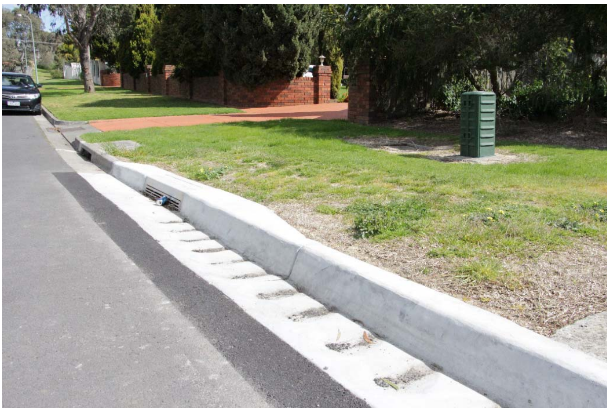
Edwin Street, Templestowe, single barrier kerb installation
