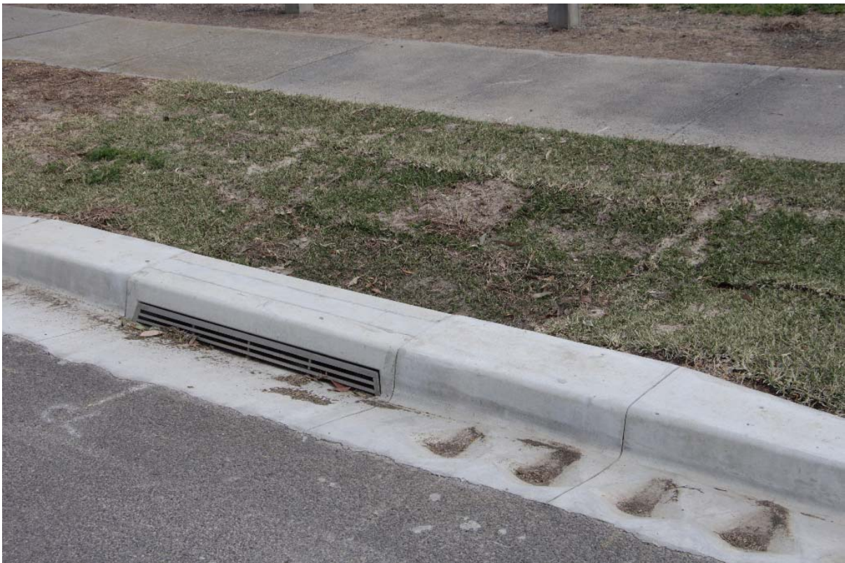
Park Avenue, Doncaster, single barrier kerb installation
