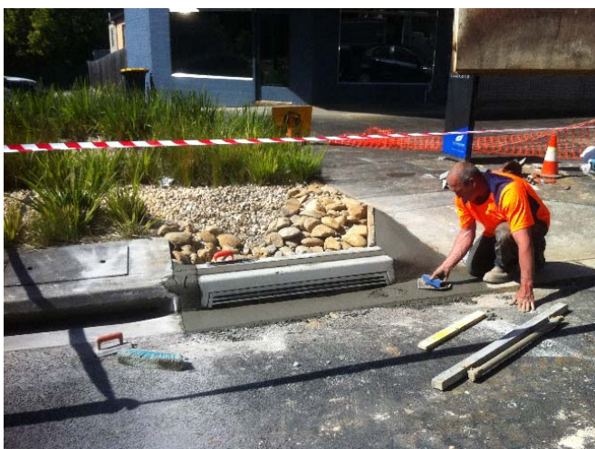
Worrell Street, Nunawading, ZAM-WSUD inlet retrofit (in construction)
