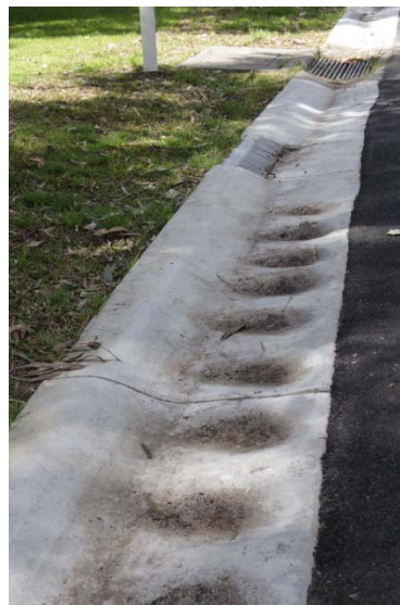
Constructed sediment grooves
