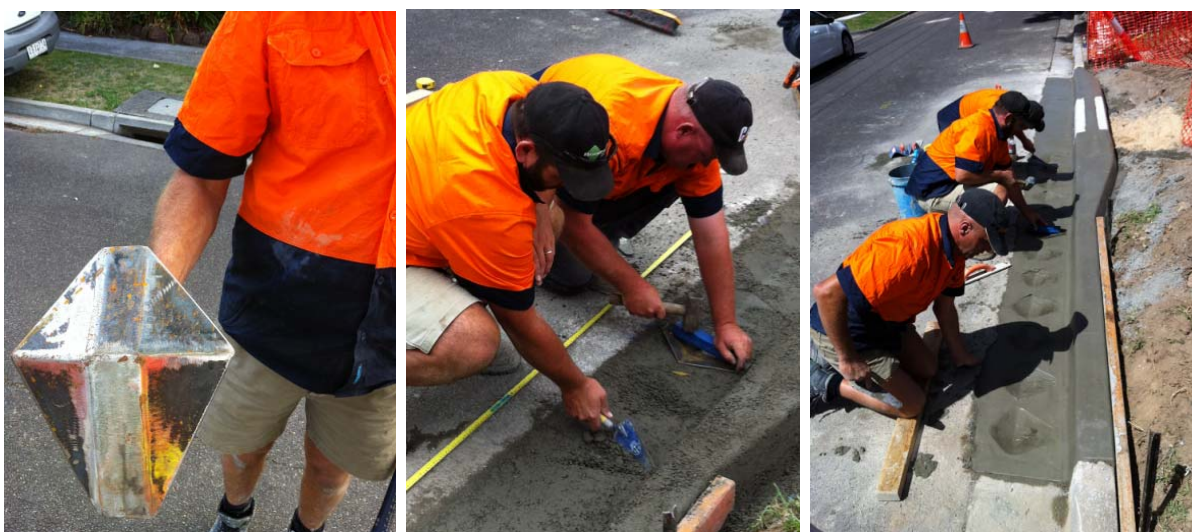
Sediment groove installation, Park Avenue, Doncaster
