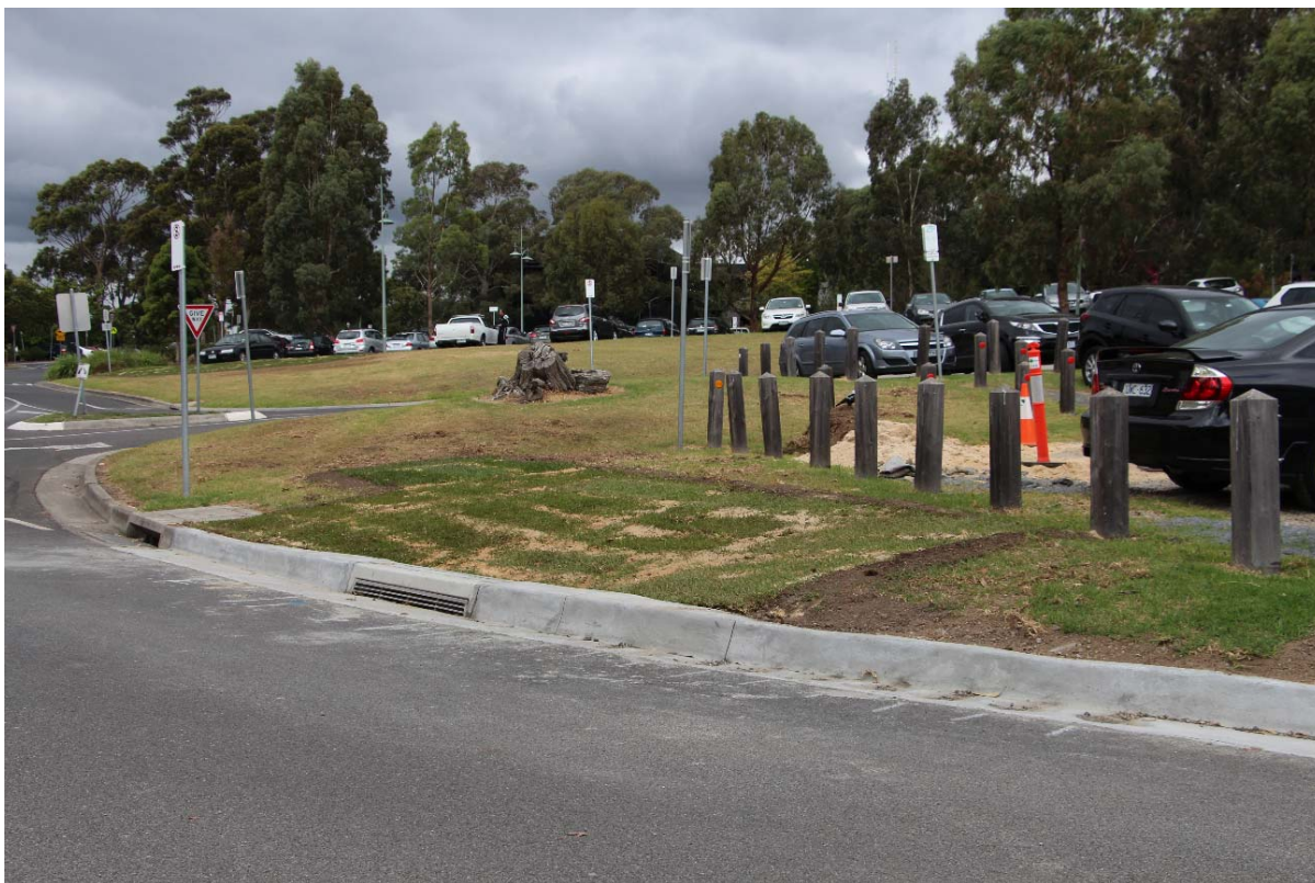
Hummel Way, Doncaster, single barrier kerb installation
